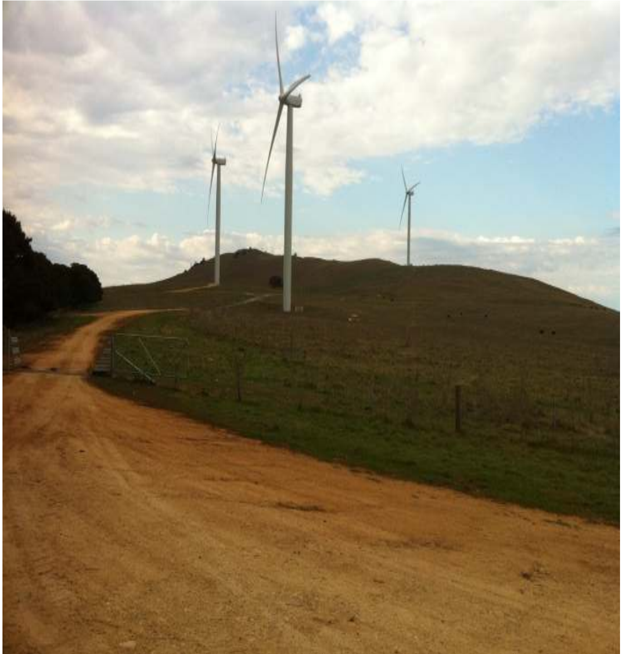
Existing Turbines, “Ellendon”, Bungendore, Capital Windfarm 1
